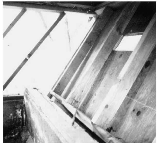
Figure 19 - This photograph shows an interior detail of a home similar to the one above, with substantial damage to a building with an unbraced tall wall.
